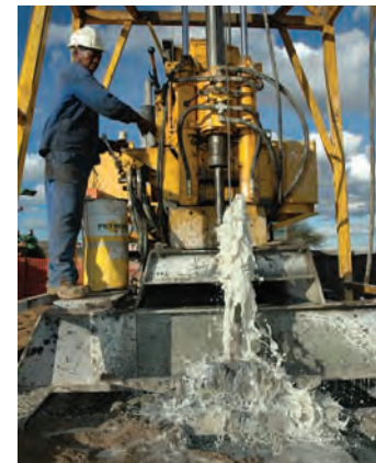
Water being used during drilling
